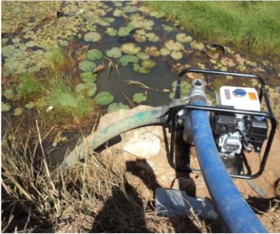
Plate VII: Pump machine in the excavated pit
