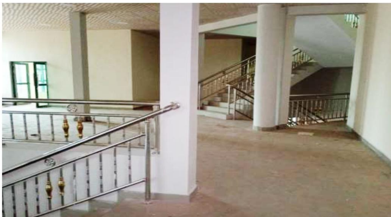
Inside the Centre
